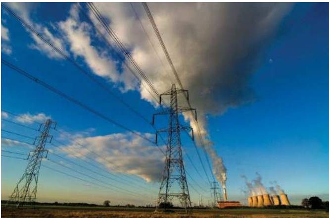
Figure 29.11 Power lines carry electricity from power station to consumer.
