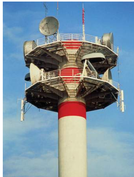
Figure 20.17 A microwave tower.
