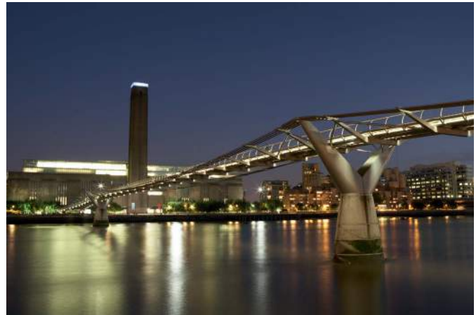
Figure 19.29 The 'wobbly' Millennium Footbridge in London was closed for nearly two years to correct problems caused by resonance.
