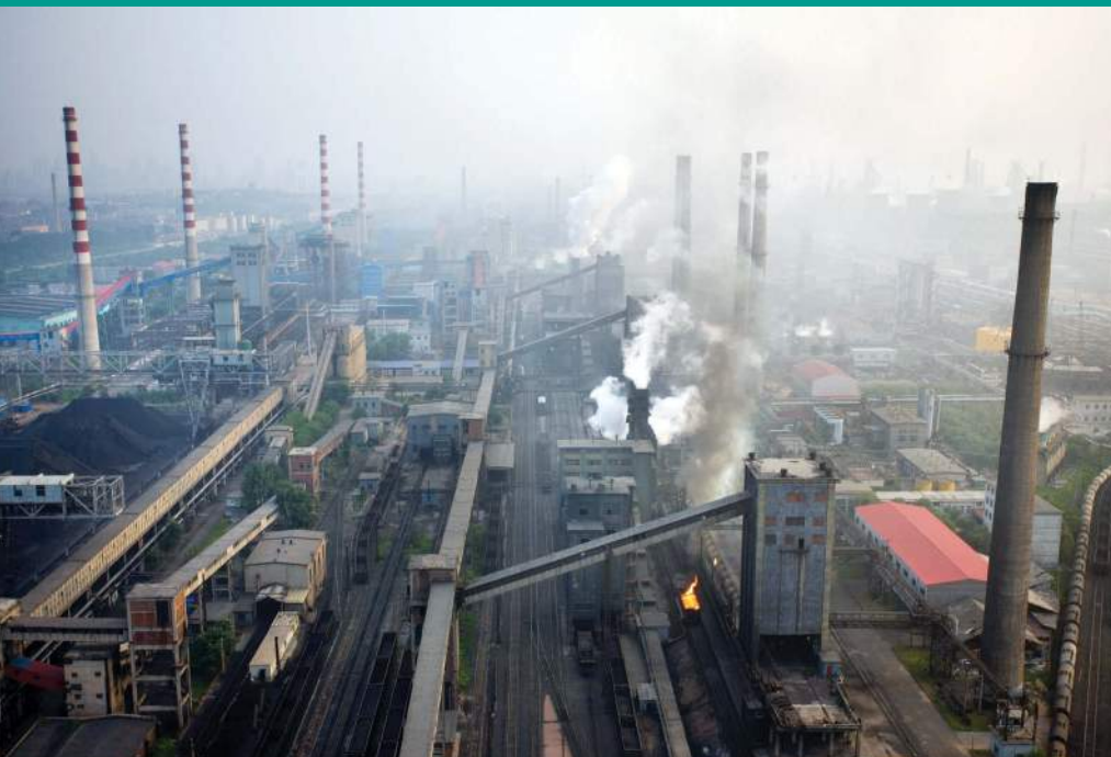
Figure 5.1 Anshan steel works, China.
