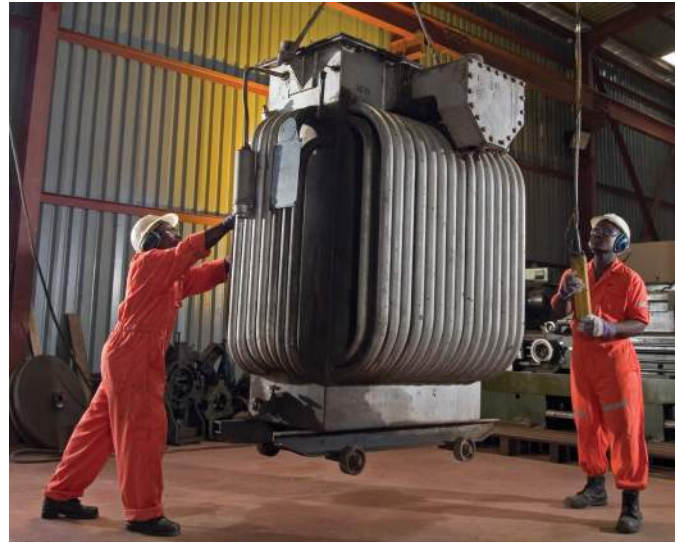
Figure 29.14 Installing a new transformer in a gold mine in Ghana.
